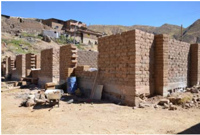
Windows removed and cracked blocks replaced, the school is ready for the geomesh. Courtesy of GHI/Stanford/PUCP
