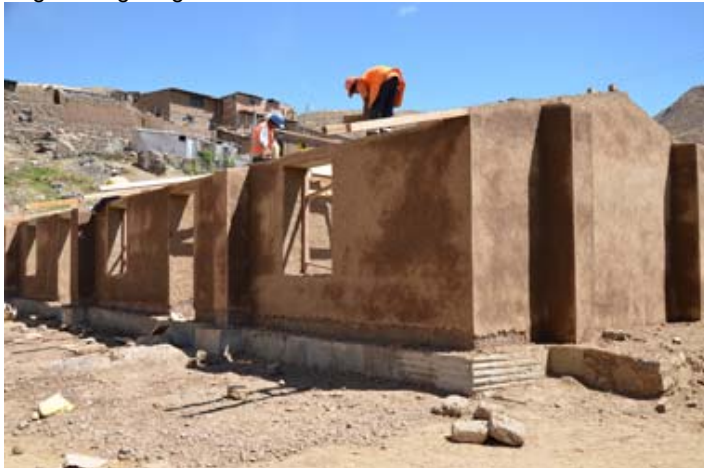
The geomesh covered, workers begin the new roof. Courtesy of GHI/Stanford/PUCP
