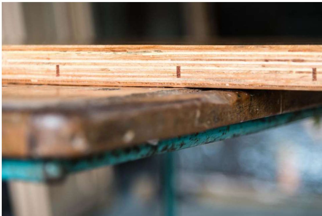
Bhutan Model tabletop edge detail. The notches are filled with small redwood pieces that have both a functional and an aesthetic role.
