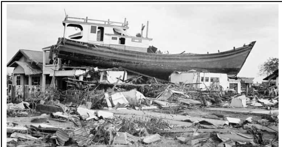
Tsunami damage in Banda Aceh, Indonesia, 2004
