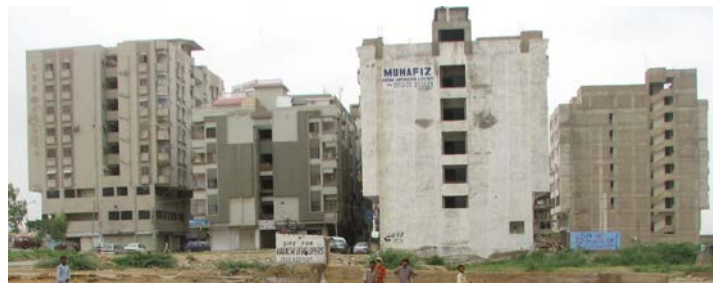
Figure 12. Mixed use and multi-family residential mid-rise buildings in Karachi, Pakistan. (Photo credit: Greg Deierlein, Stanford University)
