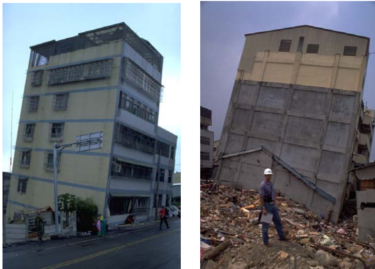
Figure 1. Collapsed concrete frame buildings in the 1999 Chi-Chi, Taiwan earthquake (Photo credits: Jack Moehle, left, and Stephen Mahin, right; courtesy of the National Information Service for Earthquake Engineering, EERC, University of California, Berkeley)
