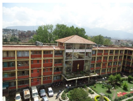
Figure 13. Hospital in Kathmandu, Nepal (Photo credit: Hari Kumar, GeoHazards International)
