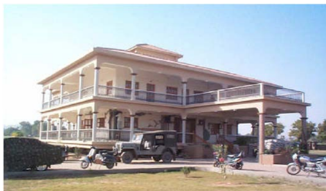
Figure 22. Infill panels provided stability to the overall structure during the 2001 Gujarat, India earthquake. (Source: Patel et al., 2001)
