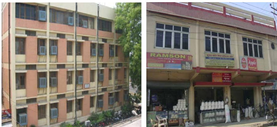
Figure 16. Commercial/office low-rise buildings in Delhi, India (left) (Photo credit: Tom Tobin, GeoHazards International); Commercial/office low-rise buildings in Dehradun, India (right) (Photo credit: Janise Rodgers, GeoHazards International)
