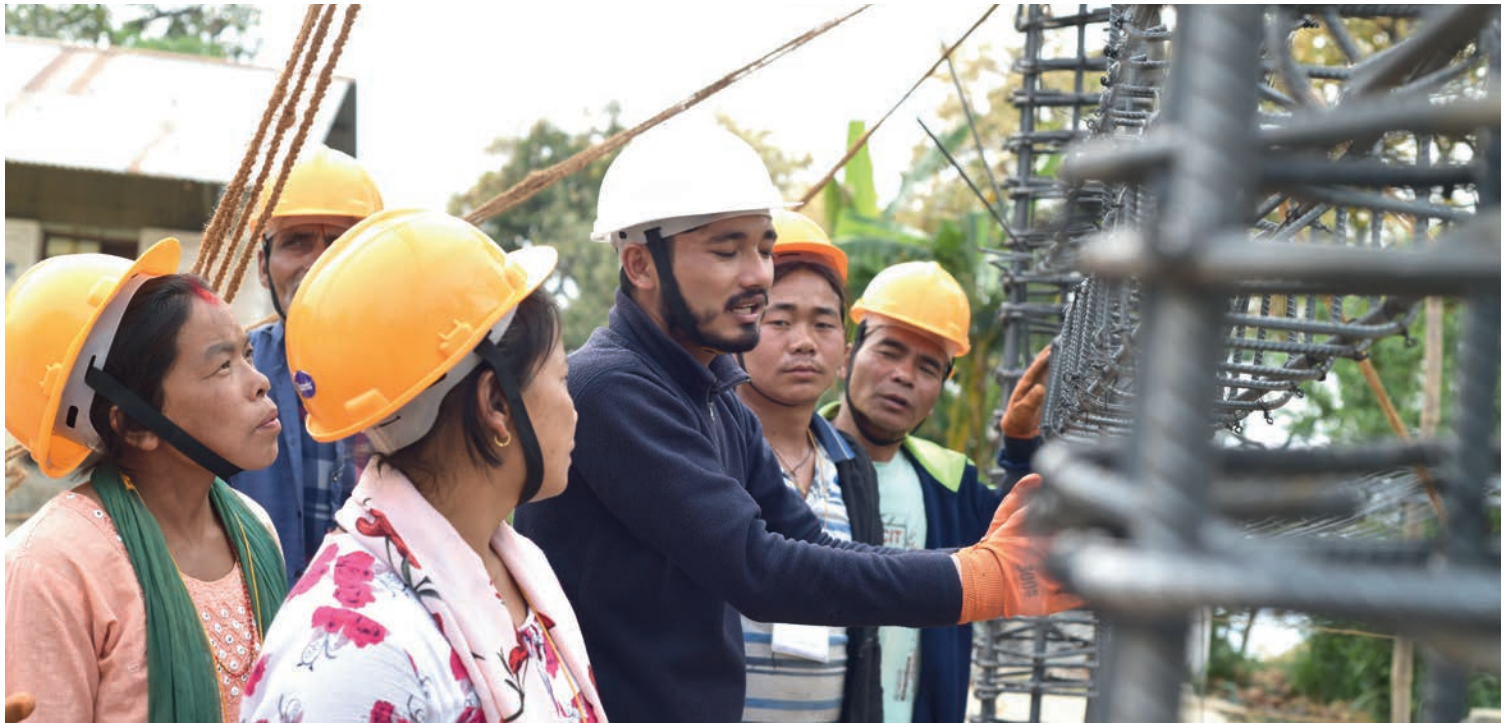
Western Nepal: Training masons, including women, on disaster-resilient construction techniques while building a school. We have been working in western Nepal since 2016 because many scientists are concerned about a future large earthquake in this particular region. The area is growing rapidly, earthquake risk awareness is low, and earthquake-resistant construction is uncommon.
